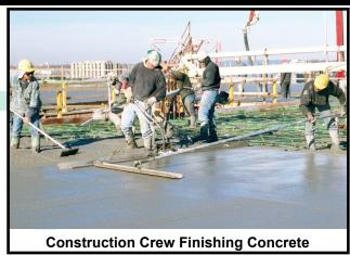
should be appropriate to placement and finishing methods, and supply should be consistent and timely. Deposit concrete as near as possible to its final location—directly from the truck chute or use wheelbarrows, buggies, or pumps. Start at the far end placing concrete abutting previously placed concrete and work towards the near end. On slopes, use lower slump concrete and work up the slope.
